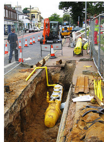
Polyethylene plastic main being placed in a trench
