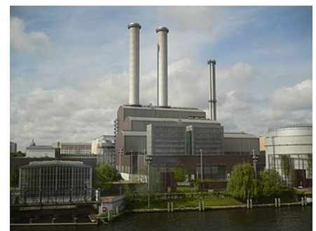
A cogeneration plant in Berlin
