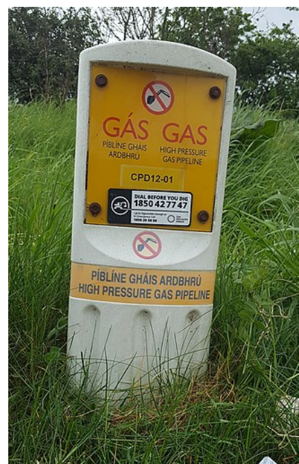
Construction close to high pressure gas transmission pipelines is discouraged, often with standing warning signs. [52]
