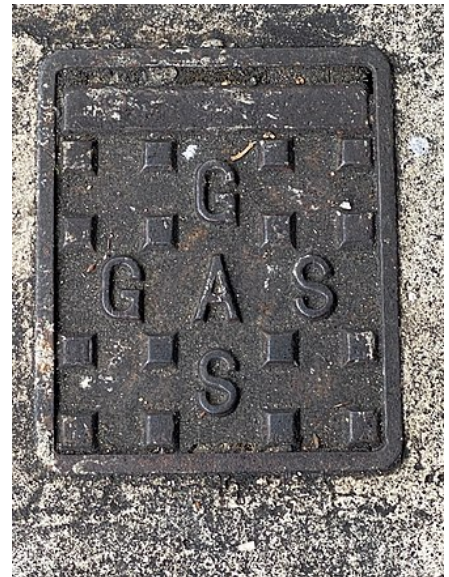
Manhole for domestic gas supply, London, UK
